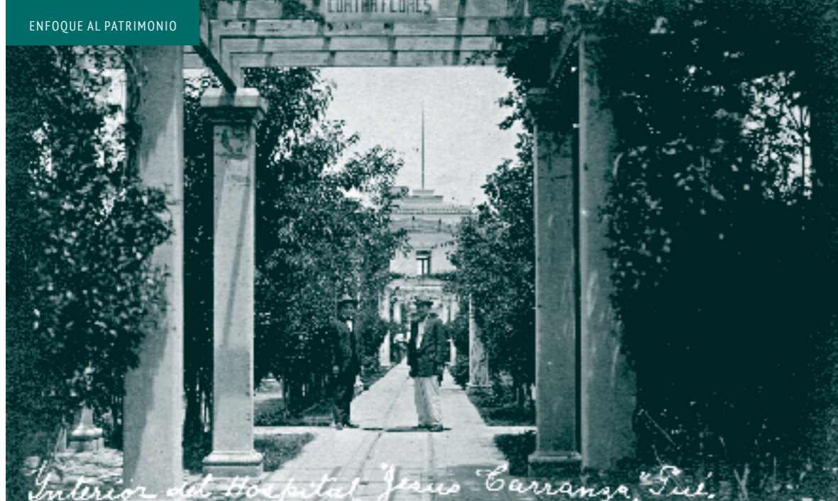
Pasillo central interior del Hospital General Jesús Carranza. Ca. 1921.
